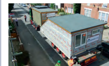
The loft components are delivered to site
