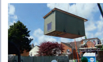
The pod is craned into place
