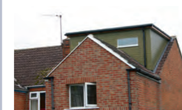
The loft is finished in just under a week
